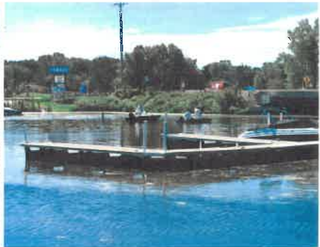
Chemical Treatment of Shallow Areas
